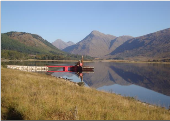
Pier for timber transshipment, upper Loch Etive Image courtesy of Isaac Forster
