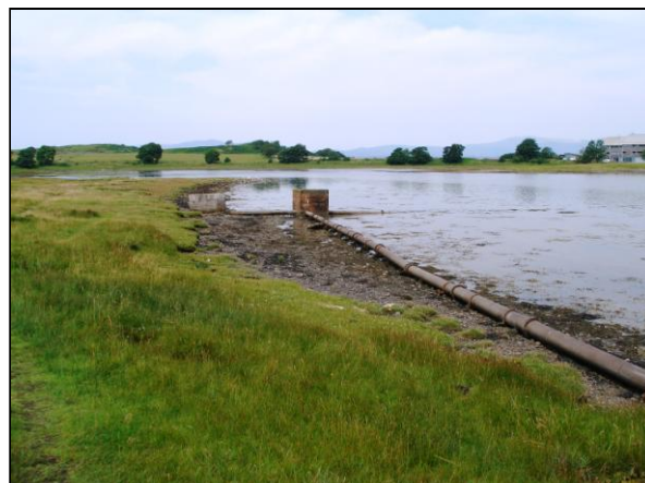
Effluent discharge pipeline at Dunbeg Image courtesy of Argyll and Bute Council
