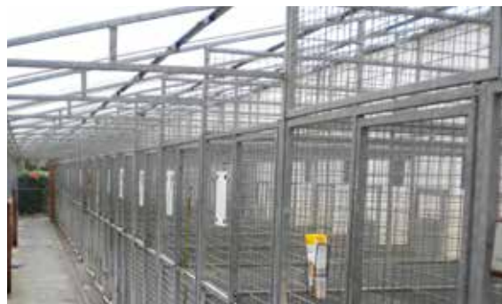
External runs protected (not full height)
