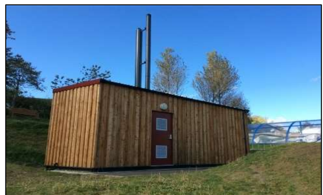
Ardrishaig Primary School biomass boilerhouse
