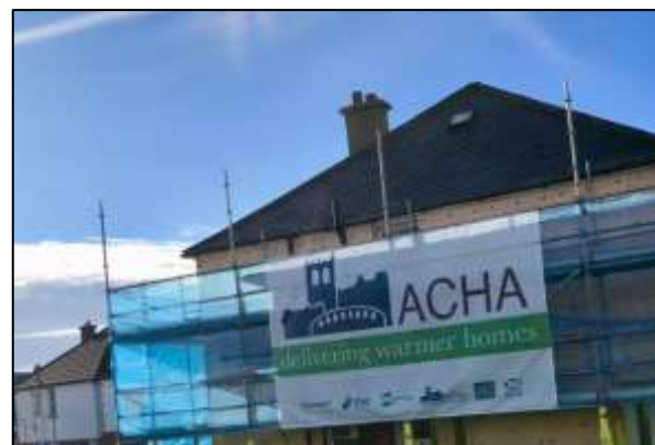
ACHA's External Wall Insulation works in Oban
