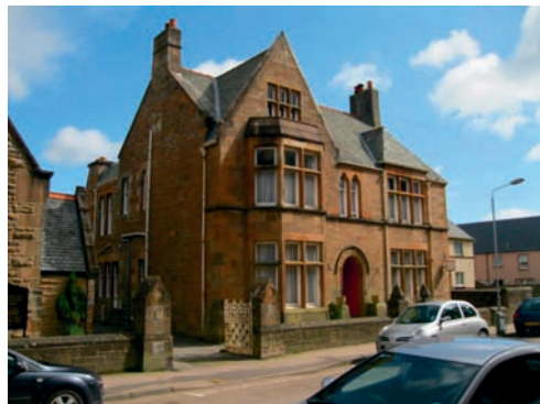
[21] The Old Rectory, Argyll Street 1885 H E Clifford 3 bay asymmetrical Tudor gothic rectory Sloping cills to windows, hood moulding over entrance door Mullioned and transomed windows Decorative wrought iron gates with a hint of art nouveau Built for the Rector of the St Kieran's Scottish Episcopal Church.
