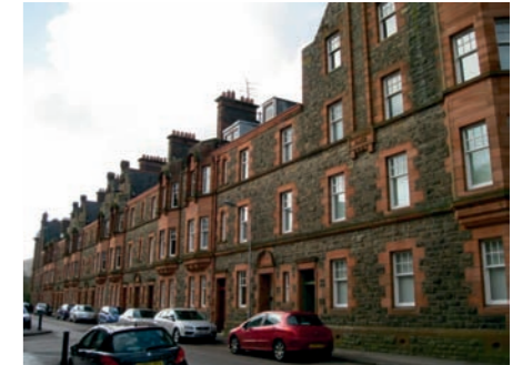
[7] Barochan Place, Argyll Street 1907 T L Watson Erected as a speculative housing venture by the architect. Watson's buildings were all designed "with conviction and impeccable taste" Bull faced stonework with sandstone dressings Corbelled bay windows Recessed columns Keystone feature projecting through open bottomed semi-circular pediments.
