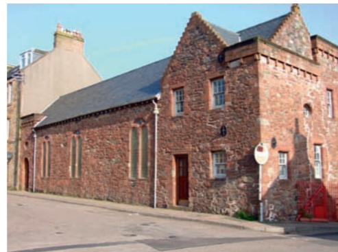
[30] Kirk Street Hall, Kirk Street 1706, restored 1904, H E Clifford Random rubble walls with dressed stone at windows Third window on left, entrance doorway and corbelled parapet at right, with crowstepped gable, all added in the 1904 restoration. Built for the Lowlanders who had settled in Campbeltown in the 17 th century. It is the oldest ecclesiastical building still in use in Campbeltown.
