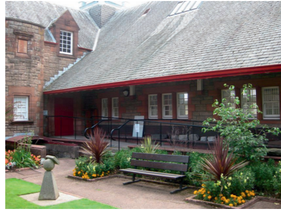
[36] Former Public Library and Museum, Hall Street, St John Street and Shore Street 1897-98 J J Burnet (Grade A listed building) Built in Free Scots Renaissance style with lantern cupola. Bull faced stonework with red sandstone dressings. Balustraded parapet. Engaged columns frame the entrance, above architraved panel and carved inscription. Art nouveau influenced iron work at entrance. Thistle motif incorporated in ironwork in Shore Street. Carved reliefs of local trades. Catslide roof in rear garden.
