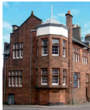
[24] The Club, Main Street 1898 H E Clifford Built with red freestone from Lochabriggs quarry, Dumfriesshire. Dressed stone and also stugged honeycomb patterned stone. High quality construction and clever use of a corner site. Semi-octagonal plain base, corbelled out at ground floor level. Ogee-roofed corner tower with dentilled cornices at eaves. Transomed and mullioned windows.
