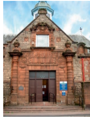
[36] Former Public Library and Museum, Hall Street, St John Street and Shore Street 1897-98 J J Burnet (Grade A listed building) Built in Free Scots Renaissance style with lantern cupola. Bull faced stonework with red sandstone dressings. Balustraded parapet. Engaged columns frame the entrance, above architraved panel and carved inscription. Art nouveau influenced iron work at entrance. Thistle motif incorporated in ironwork in Shore Street. Carved reliefs of local trades. Catslide roof in rear garden.
