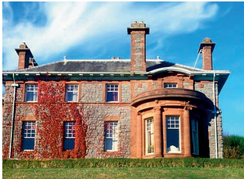
[37] Rothmar, High Askomil (Grade A listed building) 1897 J J Burnet extended 1937 2 storey, asymmetrical 4 bay American-style villa. Bull faced stonework with polished red sandstone dressings at windows. Attractive semicircular bow window with engaged Ionic columns. Built for William Broom, shipbuilder.
