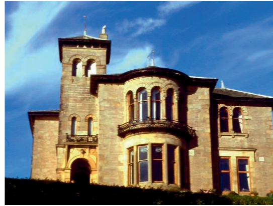
[13] Craigard, Low Askomil 1882 H E Clifford Large Italianate villa with tower and east wing. Fine bow window dominating the south façade. Arcaded windows on 1 st floor with columnar mullions and channelled vousoirs. Built for William McKersie, junior, proprietor of Lochruan distillery.
