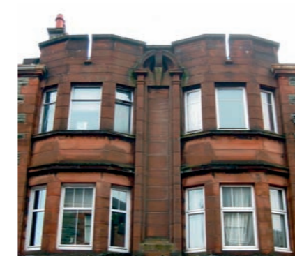
[8] Longrow South 1909 T L Watson Fine 3 storey tenement with bull faced stone work and red sandstone dressings. Circular and octagonal domed corner towers. Crenellated parapets and shallow bay windows. Keystone feature and flanking circlets in doorway lintels. Longrow South was created to sweep away the unsanitary conditions of the Wide Close which fronted Main Street.
