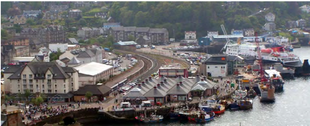
Figure 3.3 Oban Ferry and Railway Terminals (Photo source: Wikipedia )
