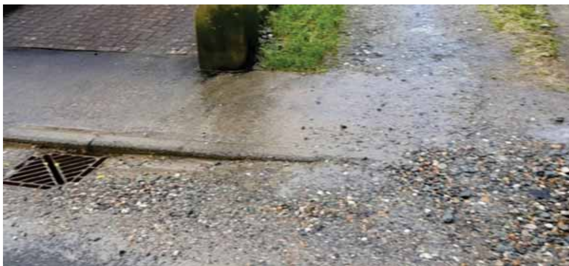
Figure 2-10: Sediment/washout from access track blocks Alexander Street road gullies in flood conditions
