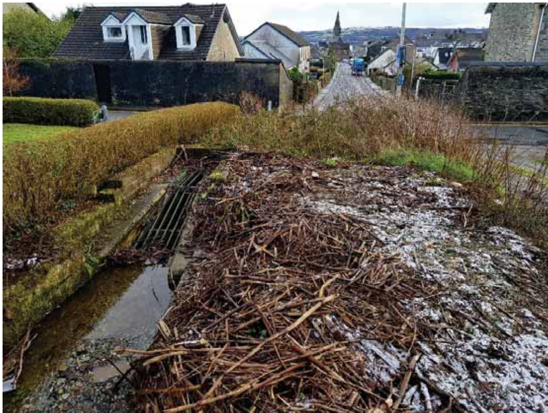
Figure 2-11: Headwall area at Alexander Street and John Street junction
