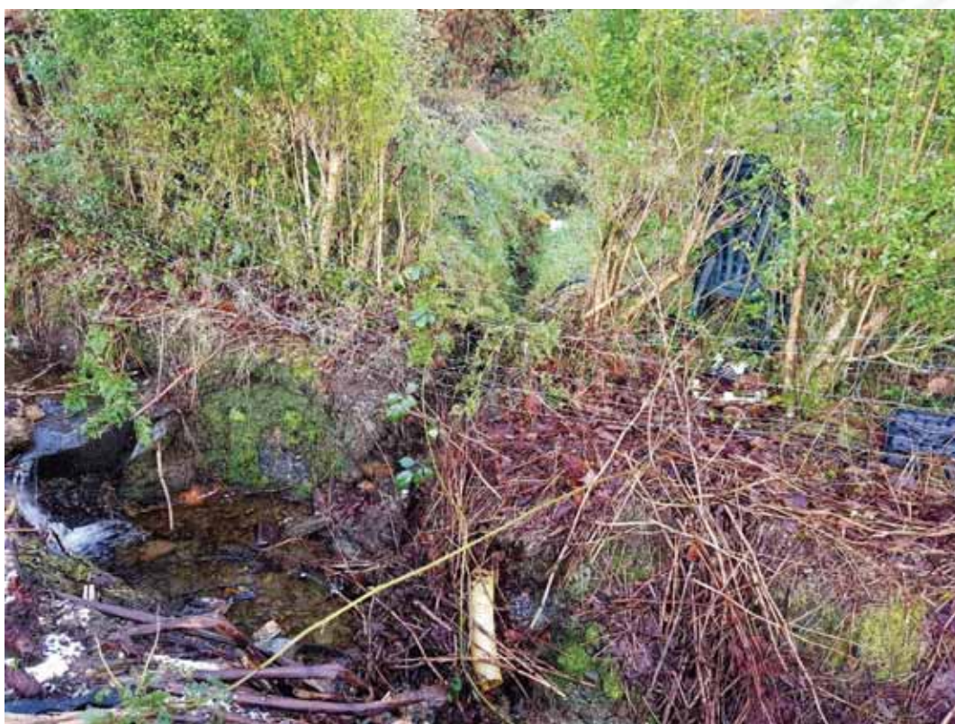
Figure 2-12: Typical condition of Channel 4 lower reach upstream of the Alexander Street headwall with informal drainage ditch from adjacent private garden
