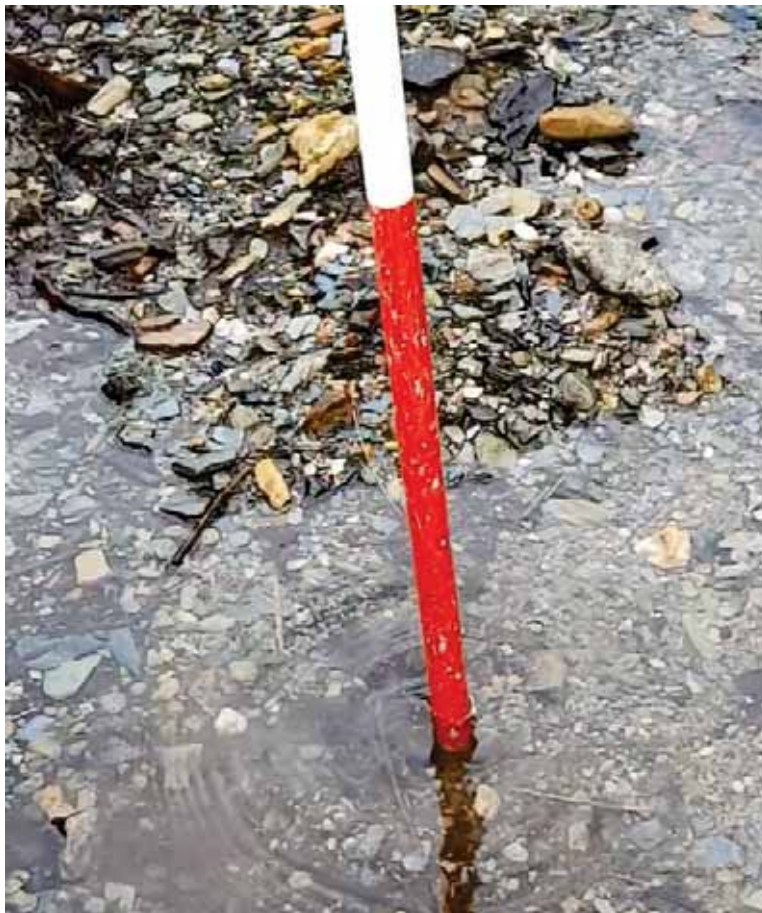
Figure 2-13: Sediment immediately upstream of headwall at Channel 4
