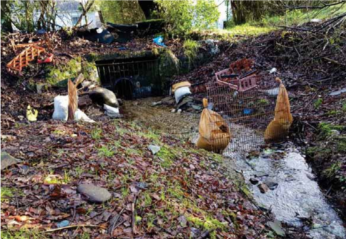
Figure 2-16: Channel 5 current headwall, screen and culvert arrangement
