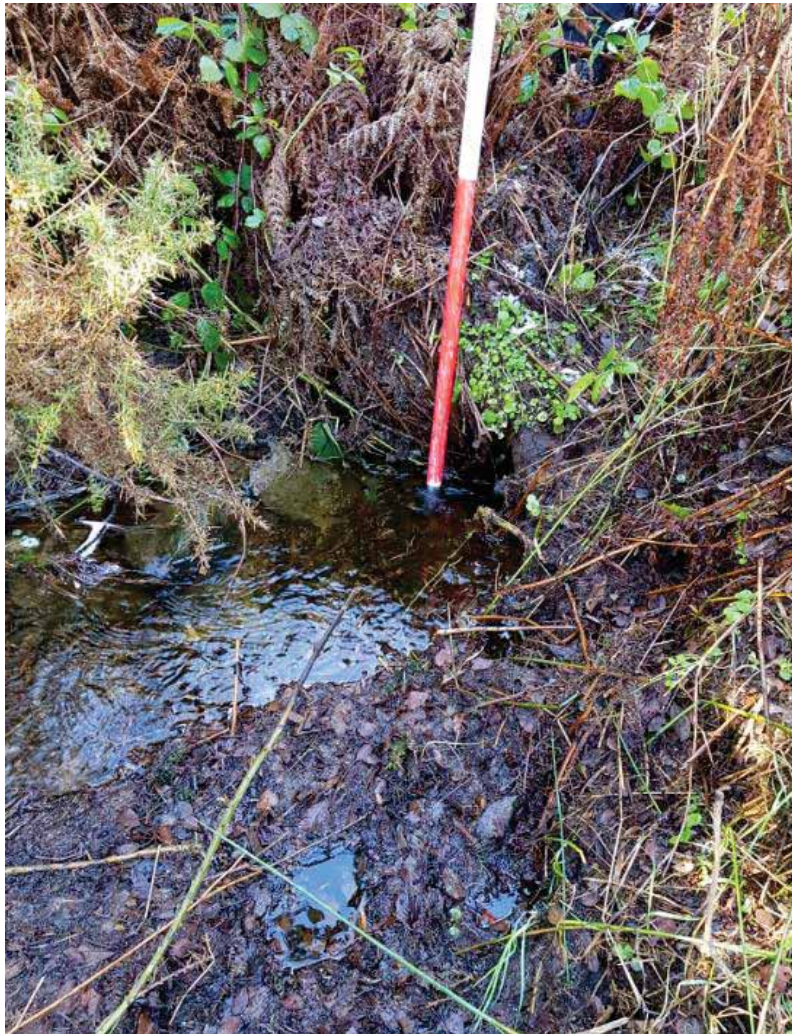
Figure 2-4: Upstream face of culvert (Channel 3)
