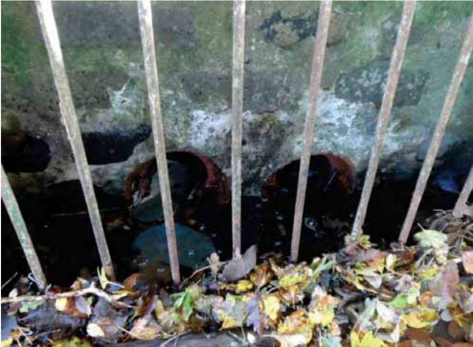
Figure 2-17: Previous headwall arrangement with 2No. clay pipes
