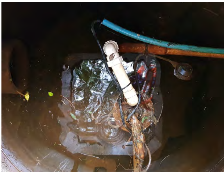
Figure 2-5: Pump (note small diameter of outgoing white pipe)
