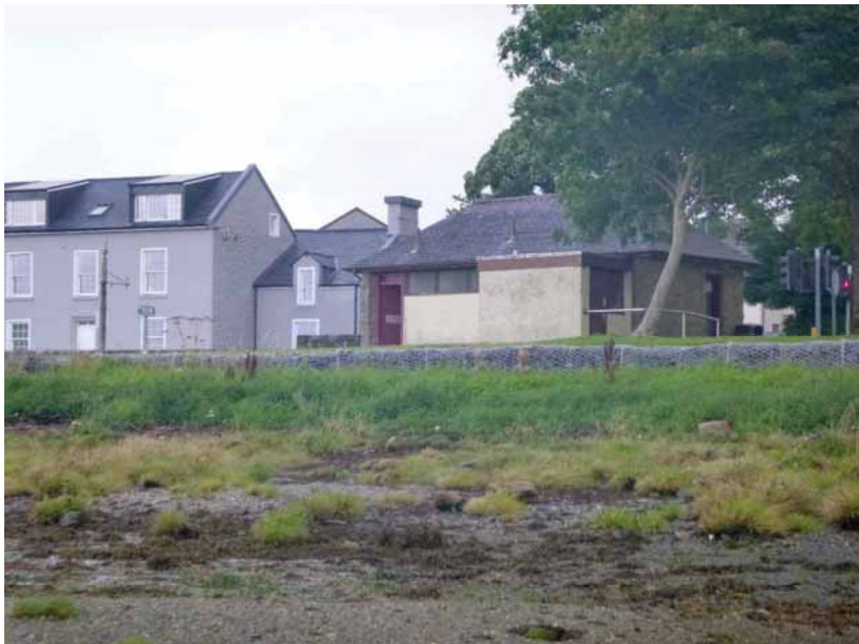
Figure 4-6: Photograph of defence within section B
