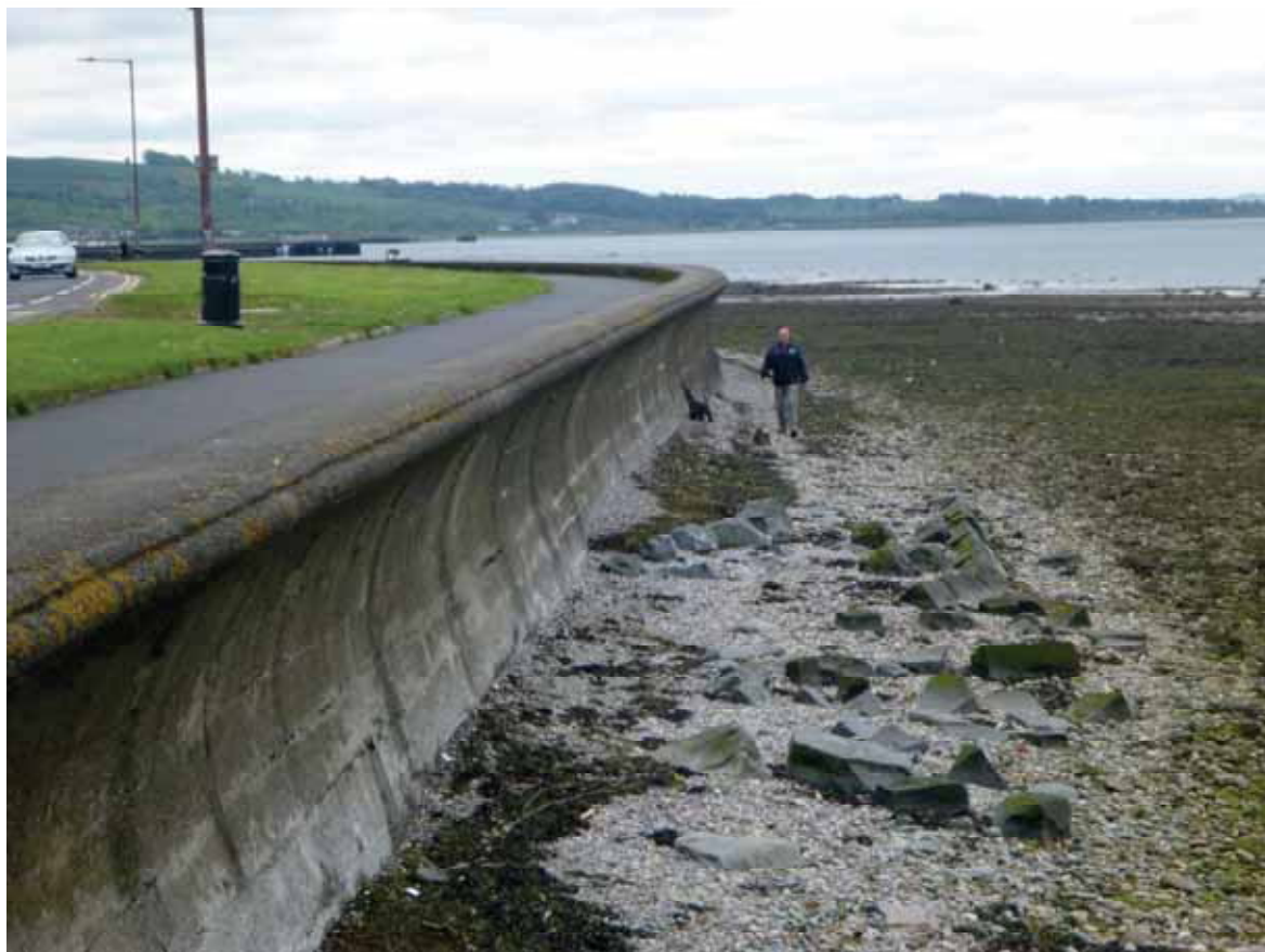
Figure 4-22: Photograph of defence within section J
