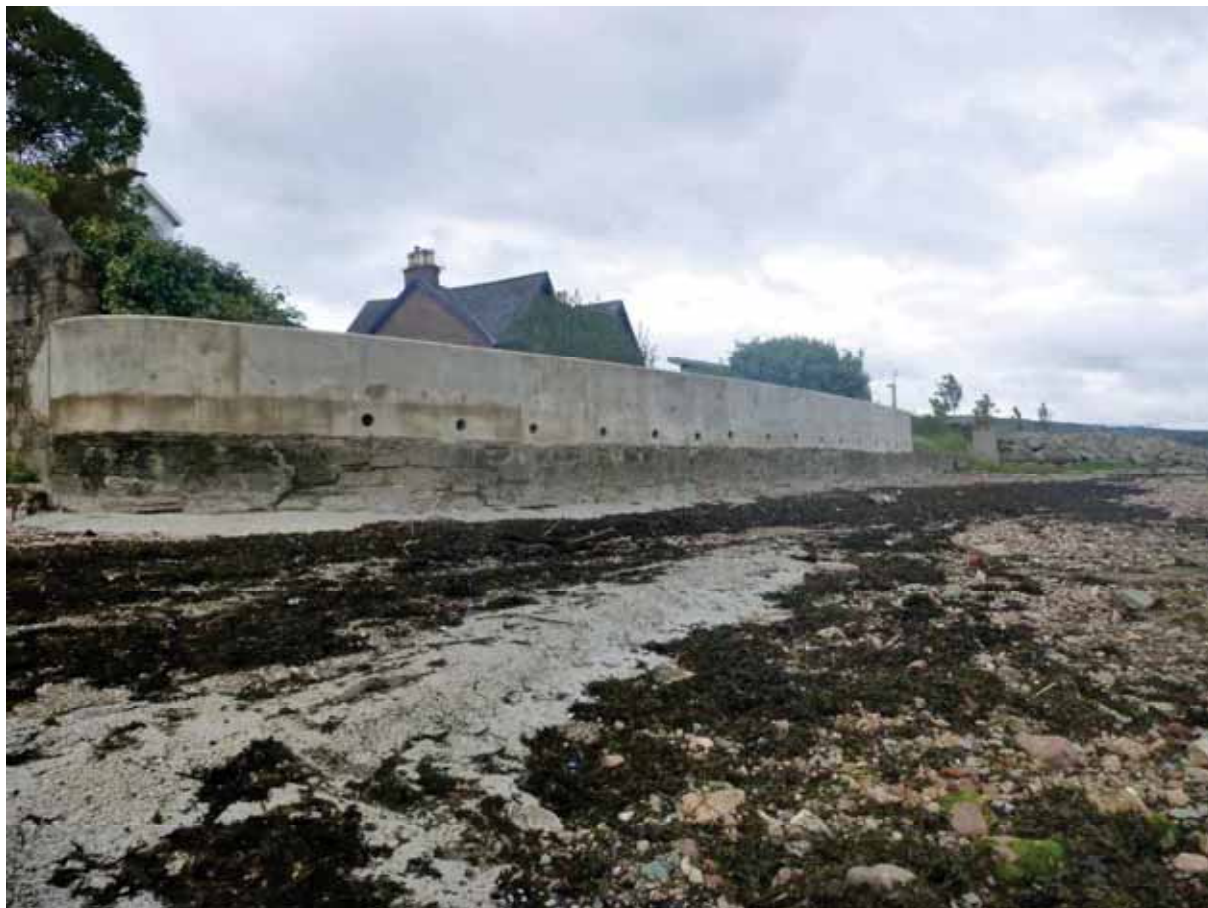
Figure 4-36: Photograph of defence within section Q
