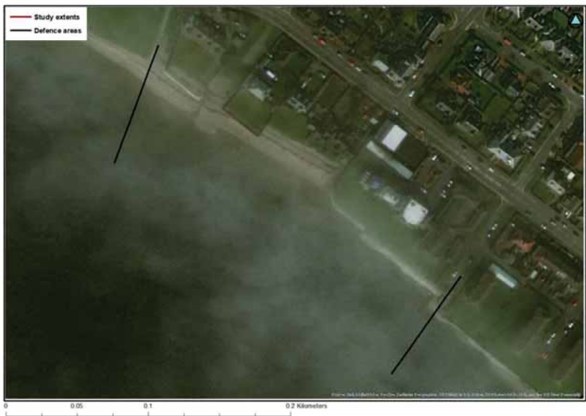
Figure 4-47: Aerial image of section V
