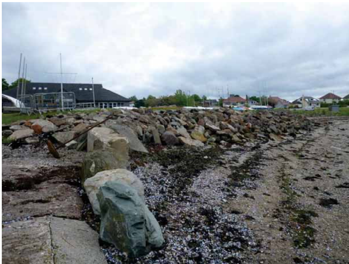
Figure 4-14: Photograph of defence within section F
