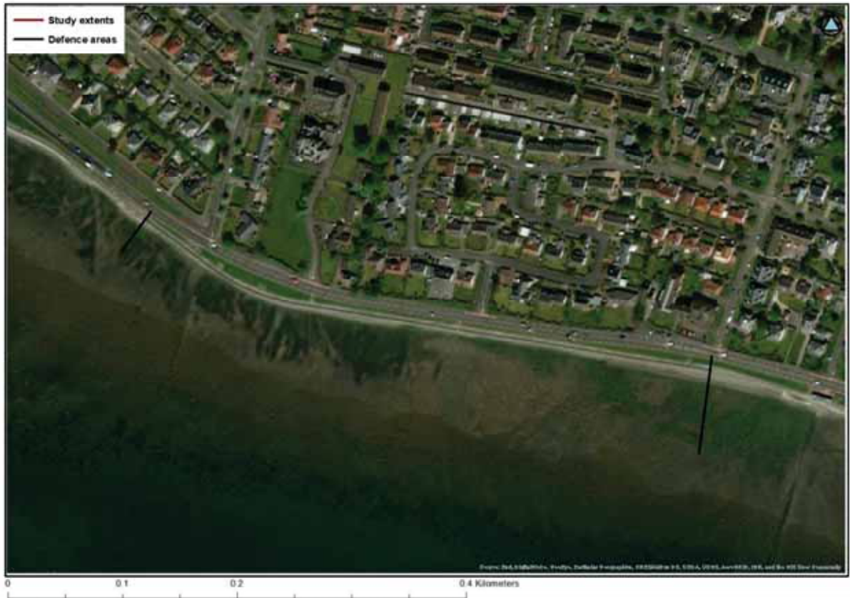
Figure 4-23: Aerial image of section J
