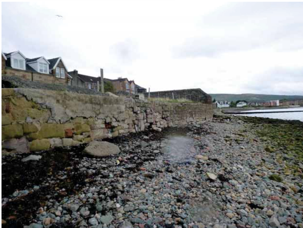
Figure 4-42: Photograph of defences within section T
