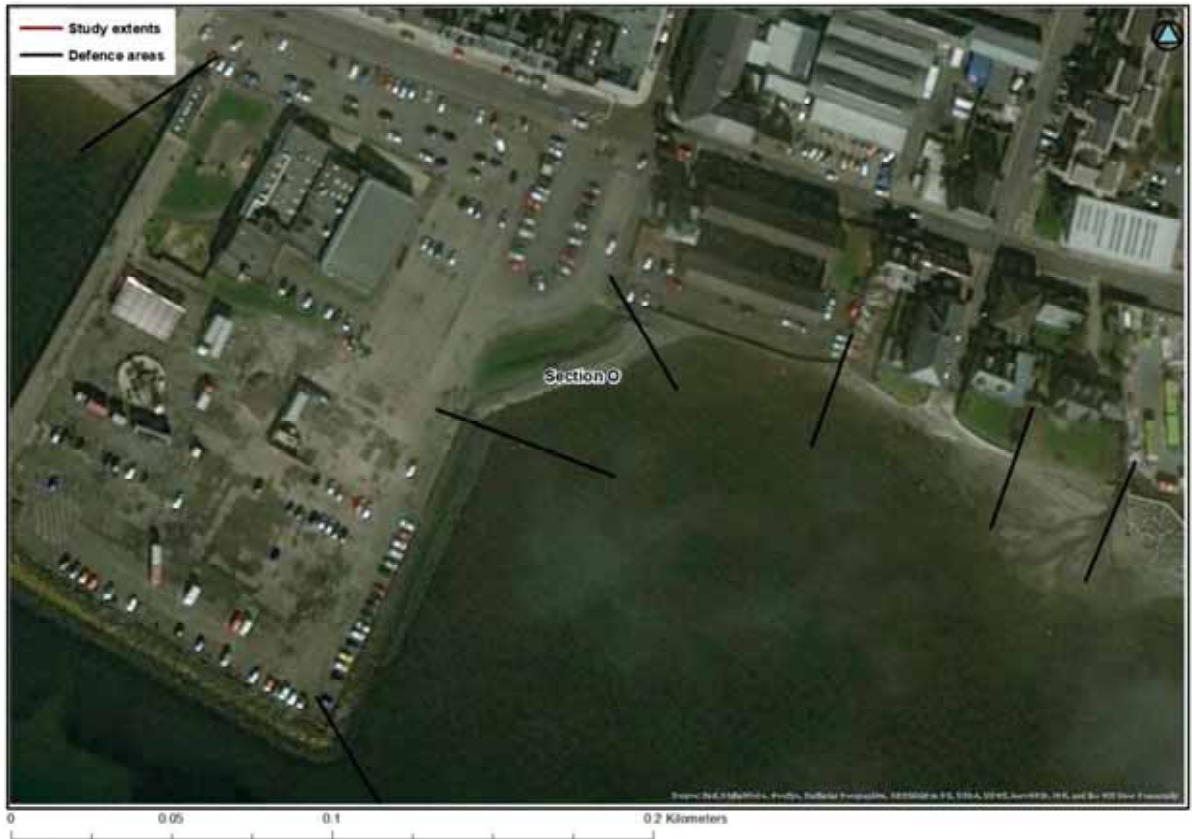
Figure 4-33: Aerial image of section O
