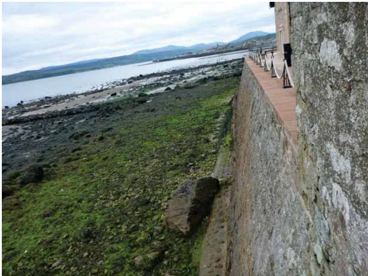
Figure 4-52: Photograph of defence within section Y
