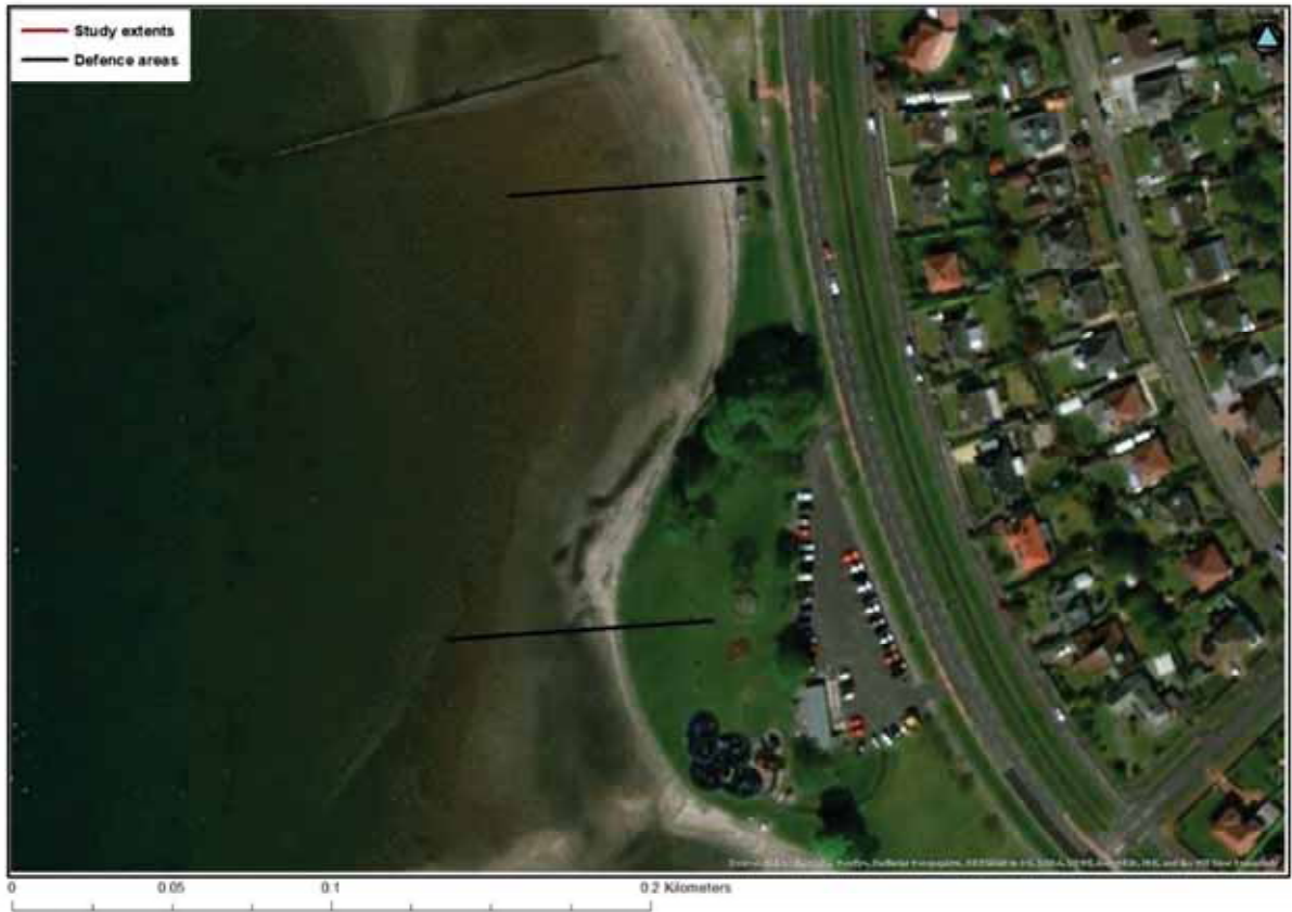
Figure 4-17: Aerial image of section G
