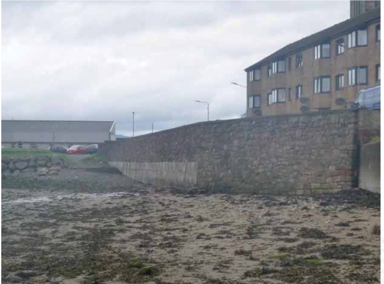
Figure 4-34: Photograph of defence within section P
