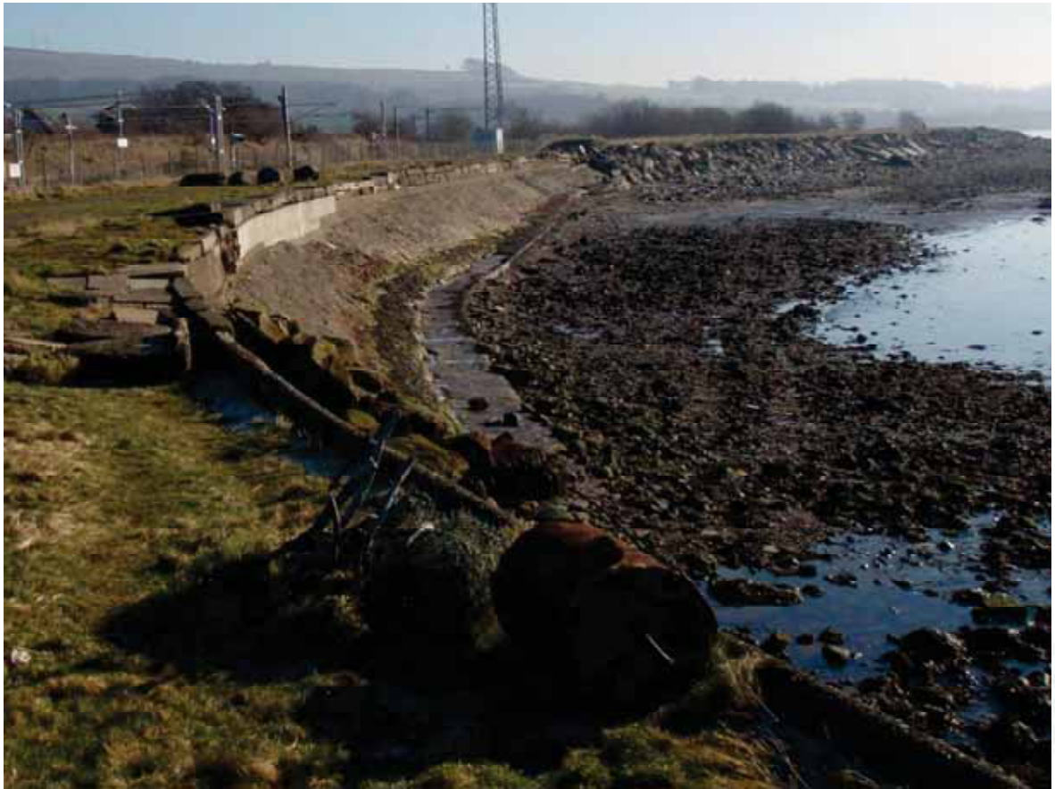
Figure 4-60: Photograph of defence within section AC
