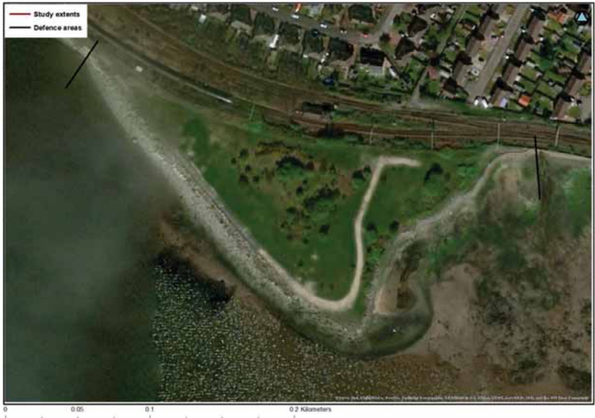
Figure 4-63: Aerial image of section AD
