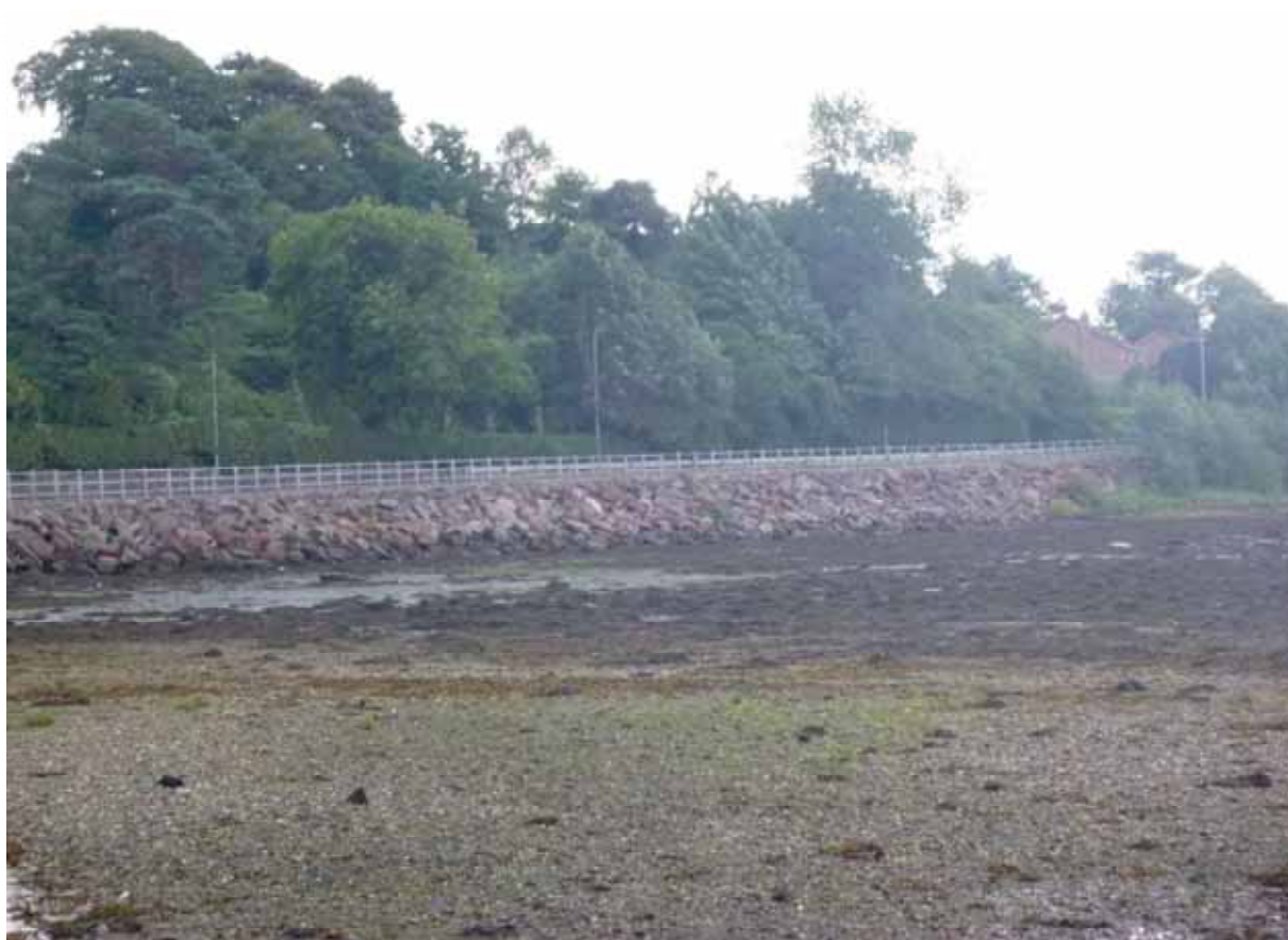
Figure 4-8: Photograph of defence within section C
