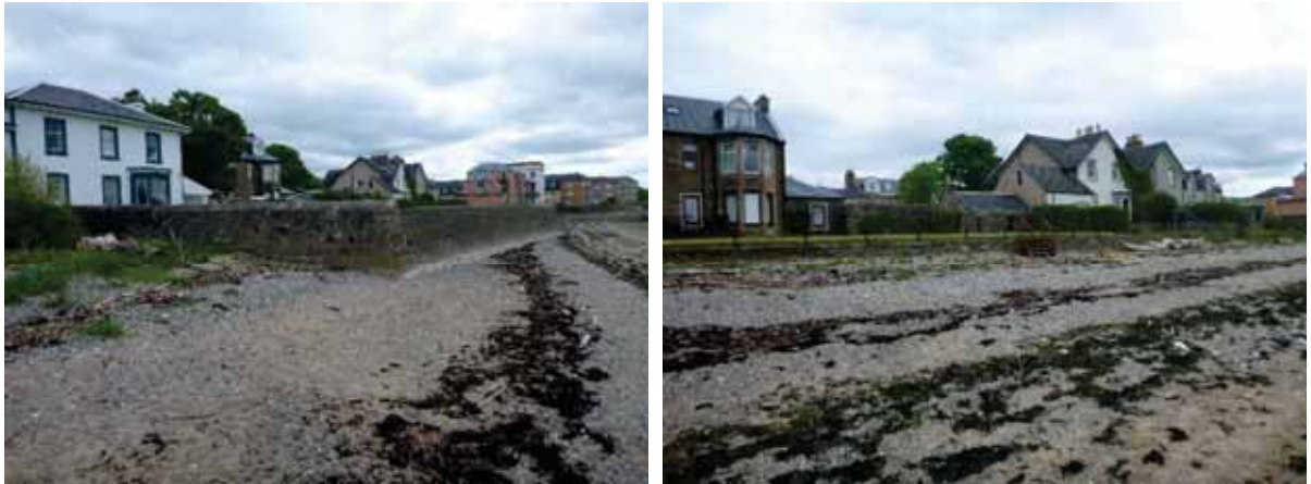
Figure 4-46: Photographs of defences within section V
