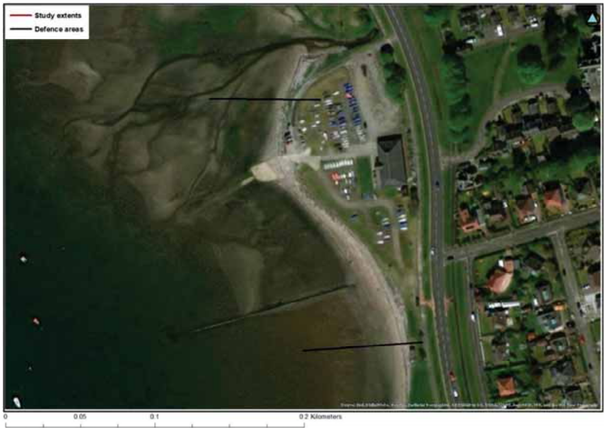
Figure 4-15: Aerial image of section F
