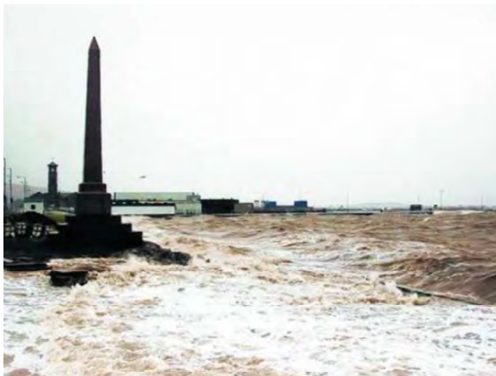
Figure 2-2: January 2014 - flooding over the esplanade at Henry Bell Monument
