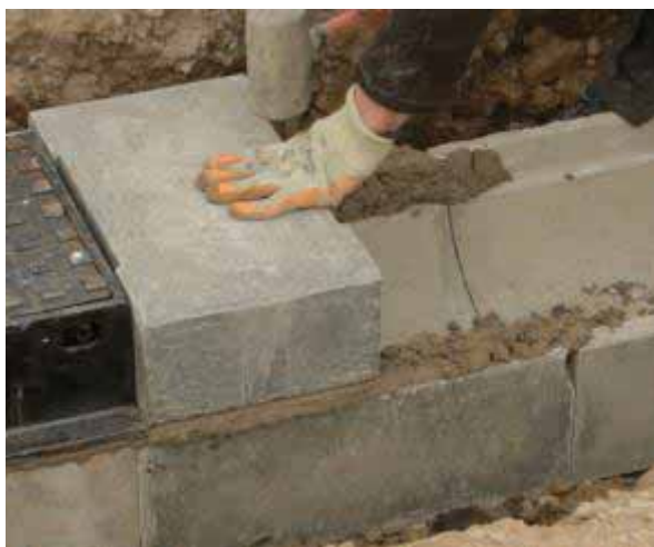
Figure 5-5: Max-E channel installation method with 365 unit
