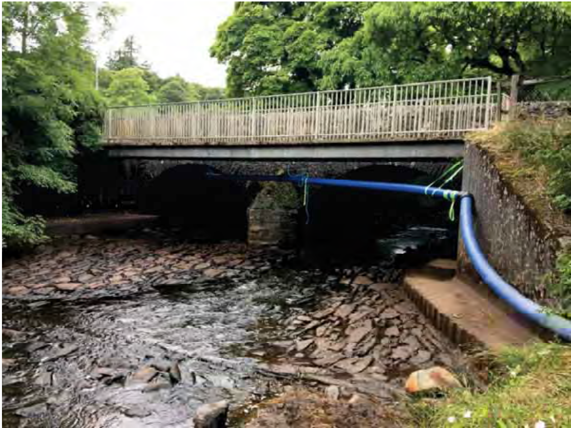
Photograph 6: Downstream of Poltalloch Road Bridge
