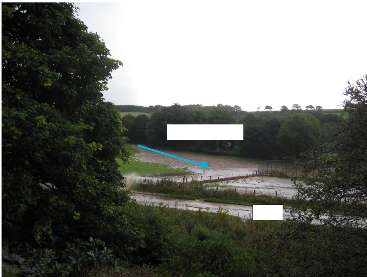
Figure 5-3 Cause of A83 flooding, August 2012 - overland flow path a)
