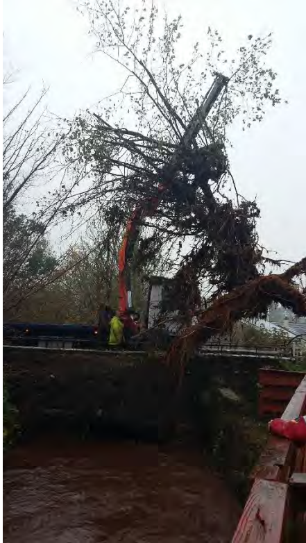
Figure 7-1 Photos of clean up following November 2015 flood event indicating blockage
