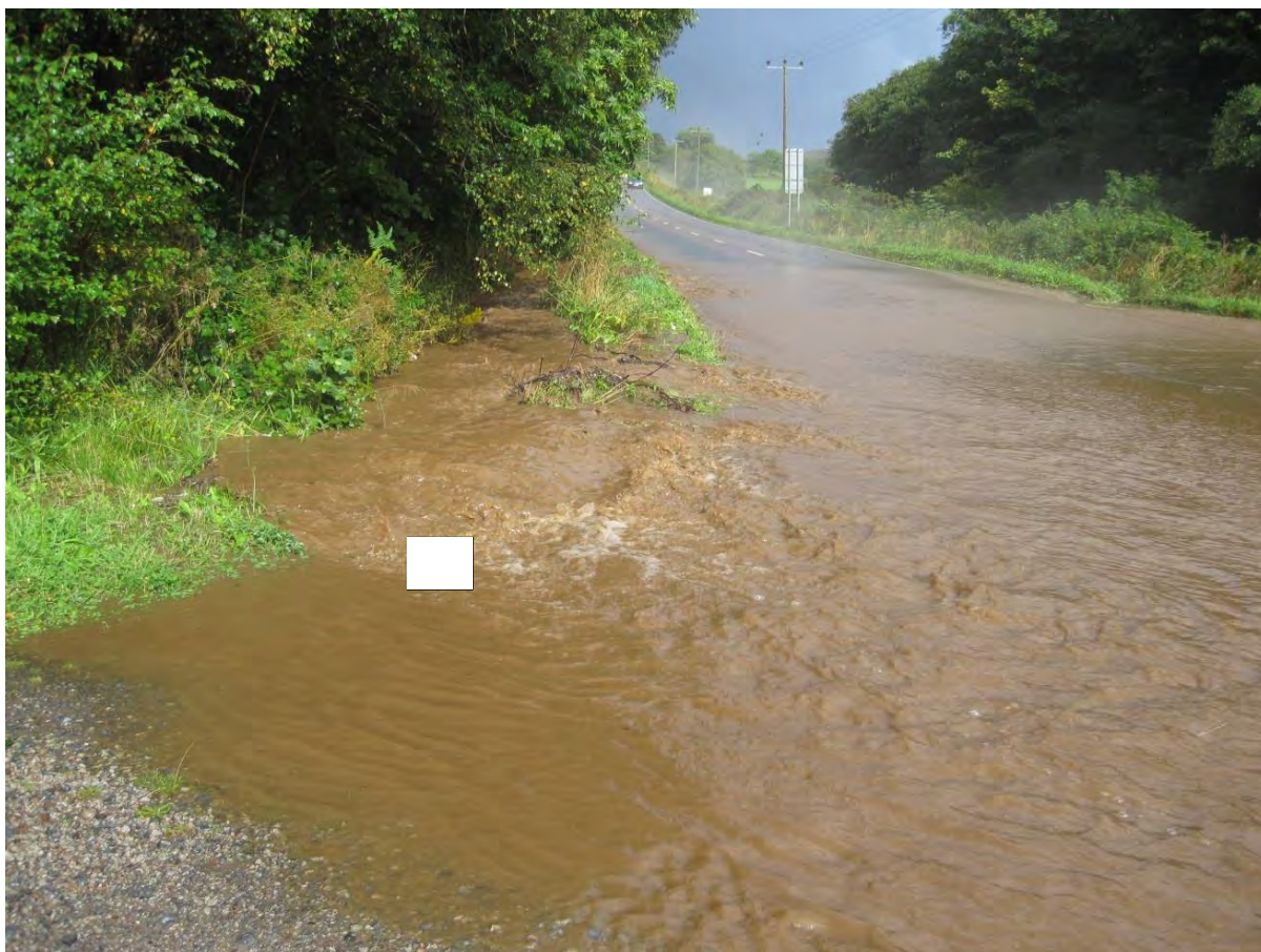
Figure 5-4 Cause of A83 flooding, August 2012 - overland flow path b)
