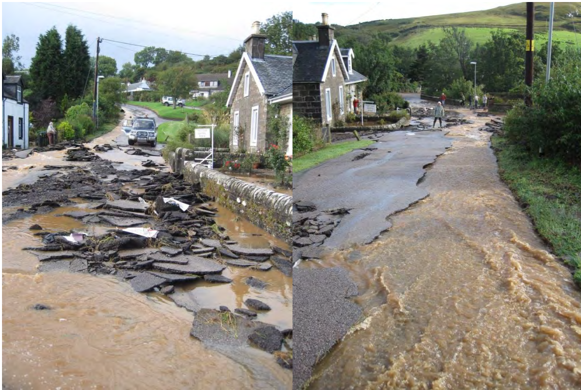
Figure 5-5 Cause of A83 flooding, August 2012 - overland flow path c)
