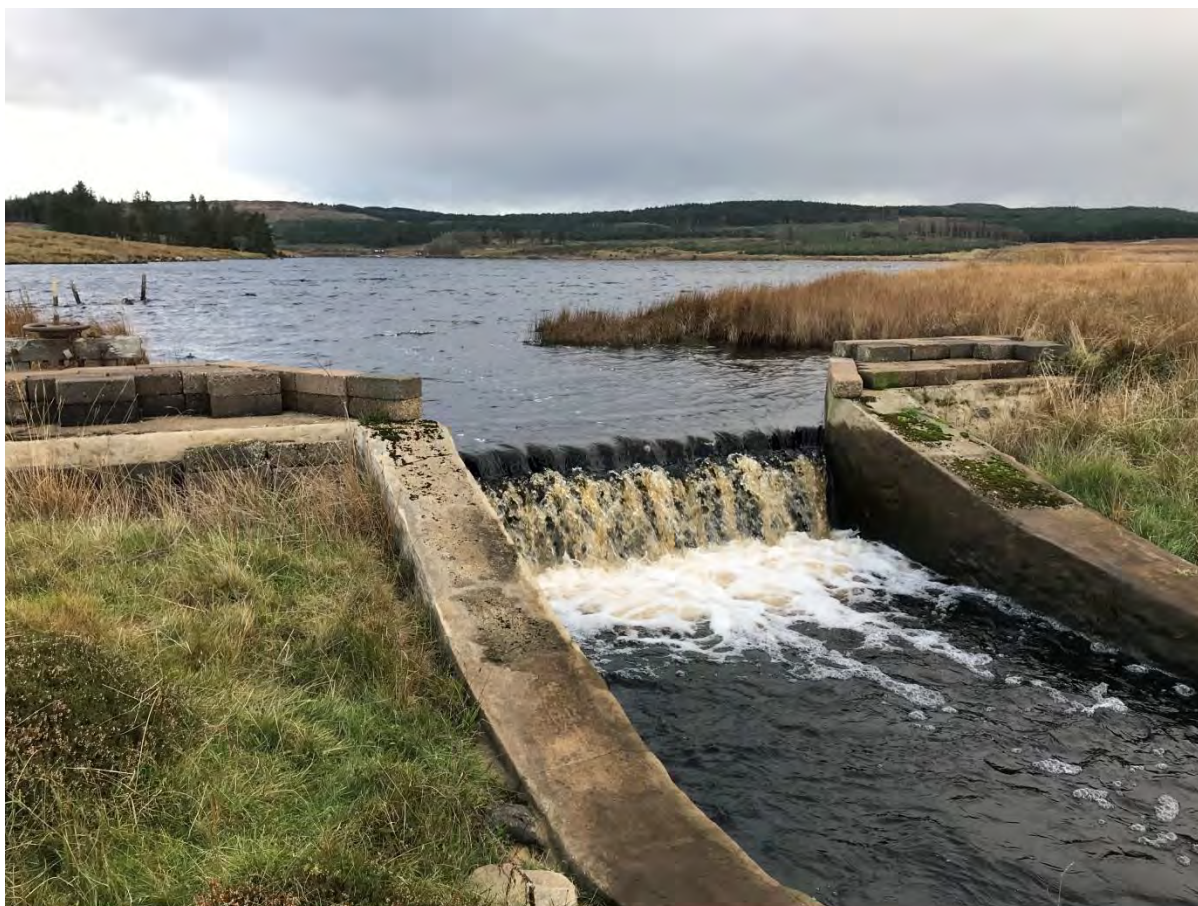
Figure 4-16 Loch Ciaran dam
