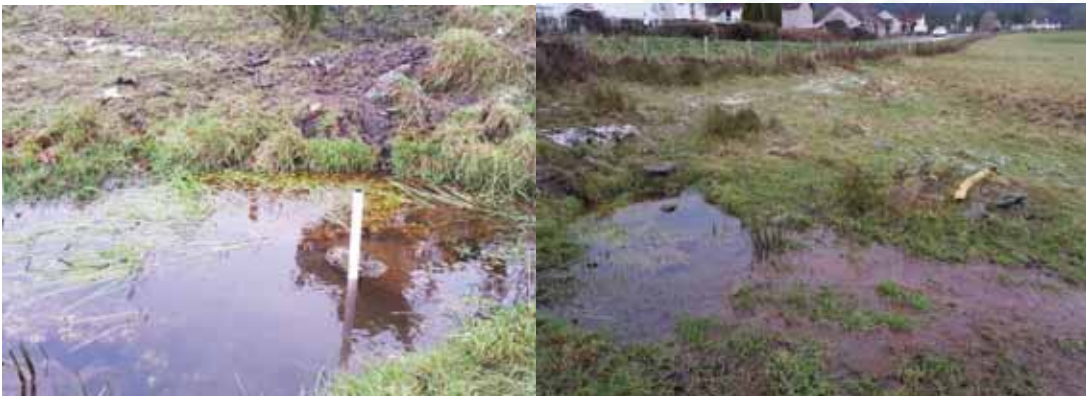
Figure 2-5: Outfall 2 from surface water drainage network fully submerged with channel infilled by silt
