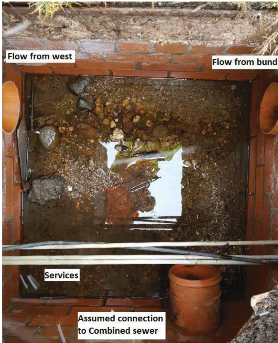
Figure 2-15: Manhole in front of house adjacent to bund
