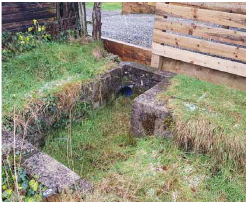
Figure 2-3: Inlet to existing drainage network on the west of the estate
