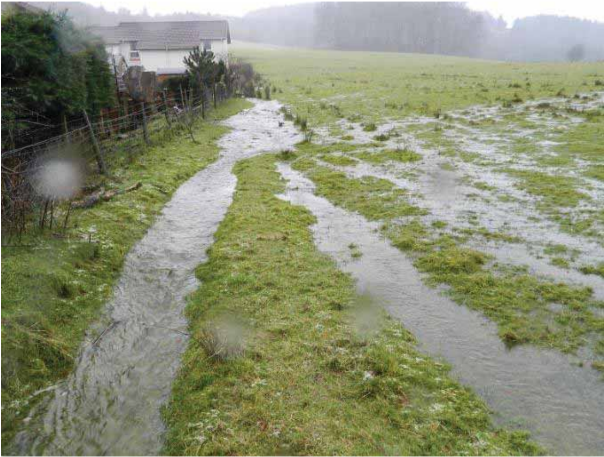
Figure 2-17: Typical overland flow paths (observed from western extent of existing embankment)
