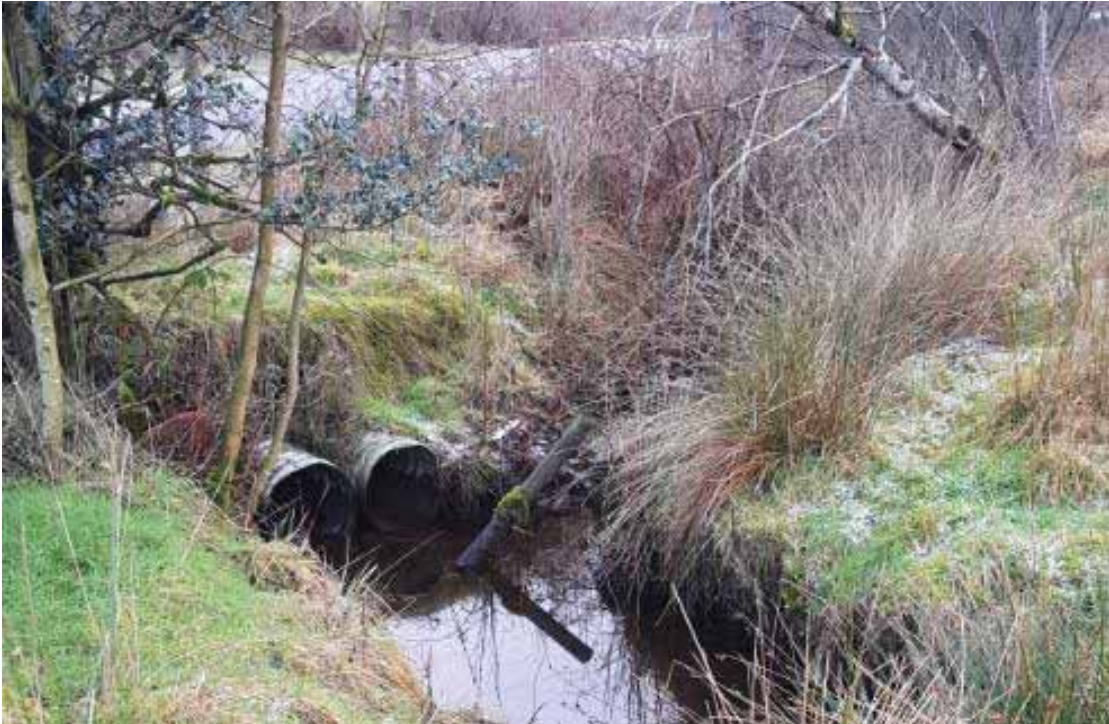
Figure 2-8: Earth mound obstructing channel approximately 5m downstream of culvert
