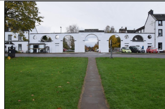
After work completed
