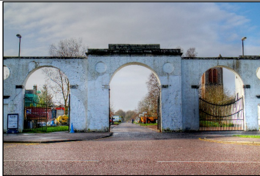
Before work started
