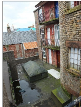
Rear deck – Before
