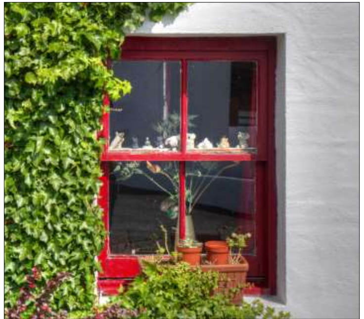
Traditional sash and case window with slim astragals—an asset to the conservation area
