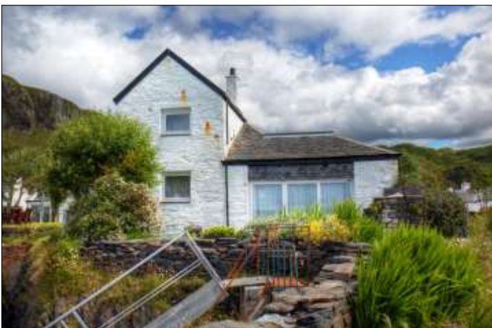
The former Engine House
