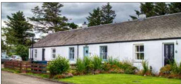
New, inappropriately small, chimneys
