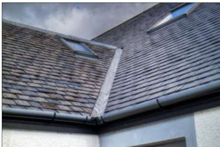
New and reclaimed slates on Community Centre
