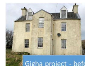
Gigha project - before
