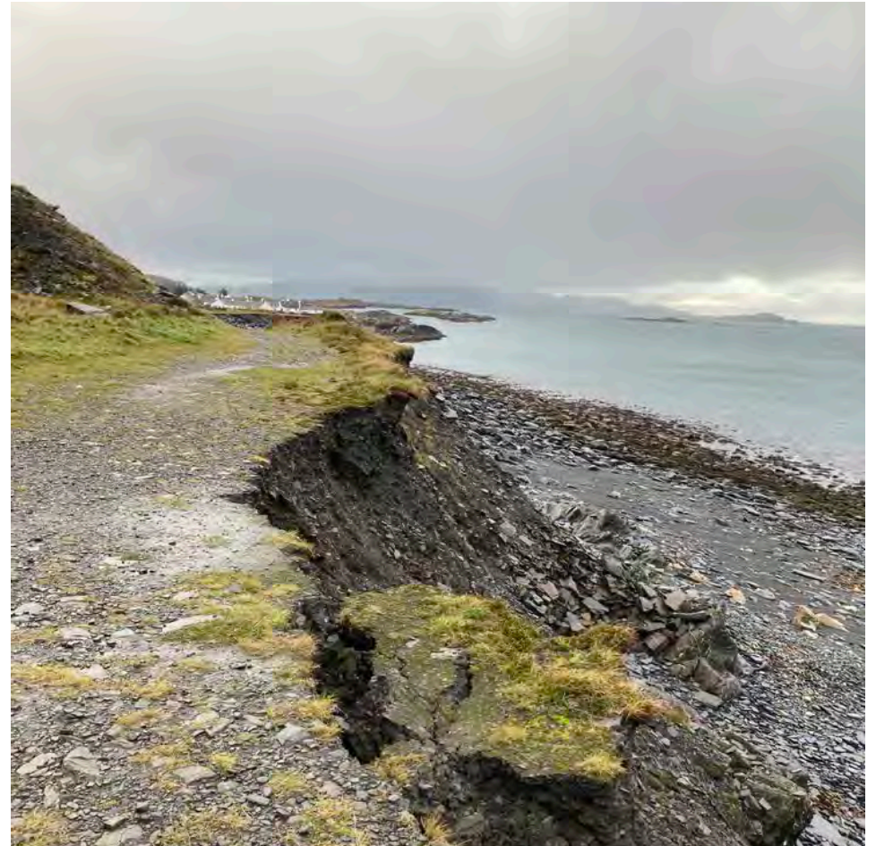
Coastal erosion, Cullipool
