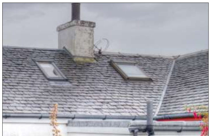
Contrasting rooflights, demonstrating how the low profile and slenderness of that on the left is more sensitive to the character of the area
