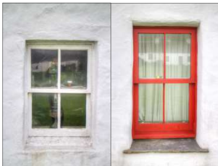
Traditional style sash and case windows—no horns, no trickle vents, suitably slim astragal
