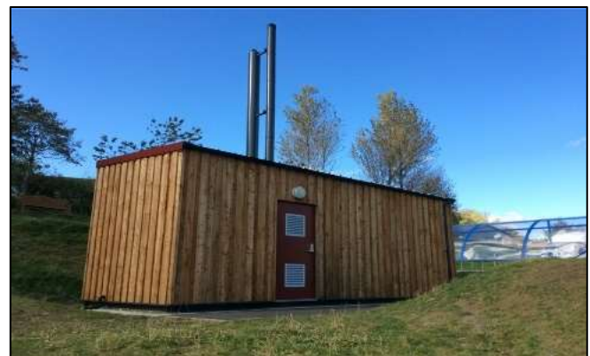
Ardrishaig Primary School biomass boilerhouse
