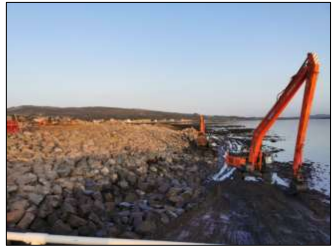
New flood defences being installed at Helensburgh Waterfront, October 2020
